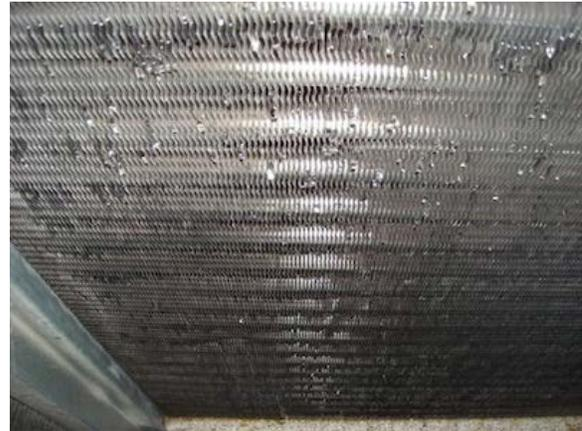
Fig 35. Forced condensation for dehumidification at an evaporator coil within an air conditioning unit
